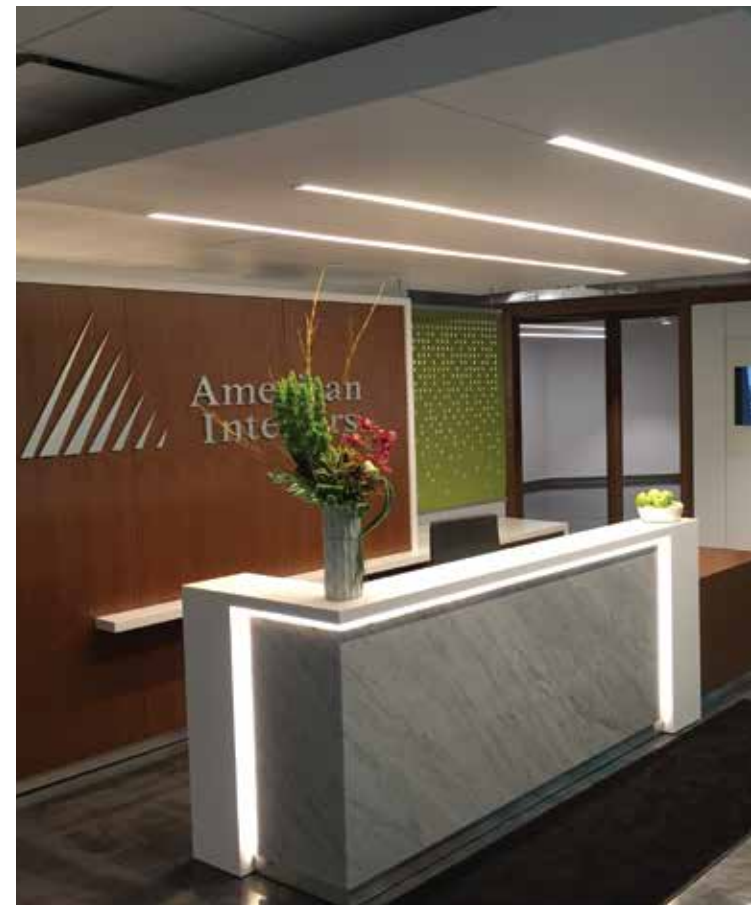
MARBLE, SOLID SURFACE, ACCENT LIGHTING, VENEER WALL
